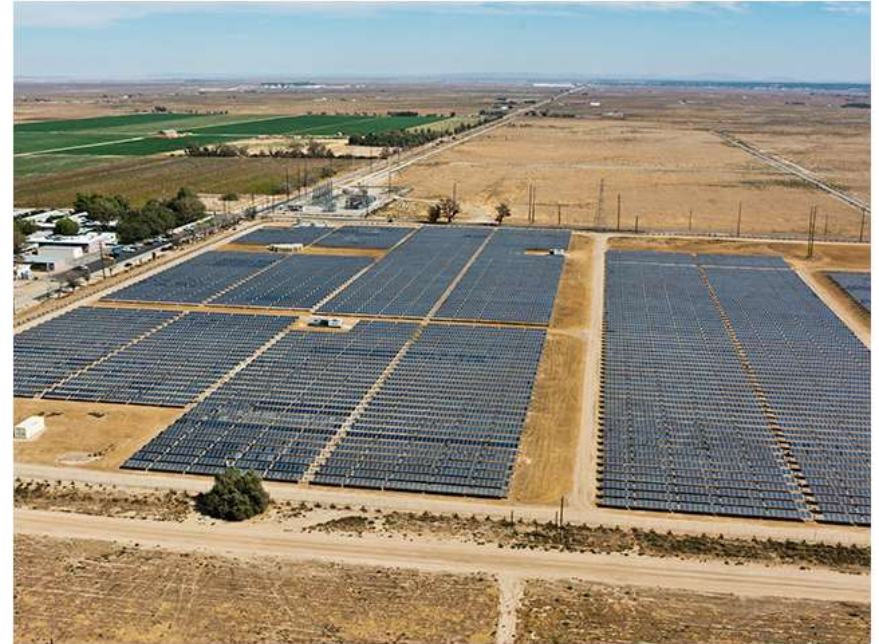
Lancaster Dry Farm Ranch, Lancaster CA Source: sPower
